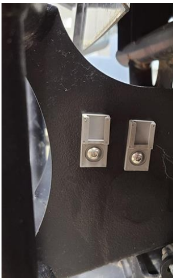
Figure 19: Mounting Storage Cap Plates
